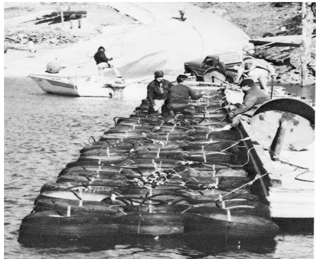
The first breakwater
