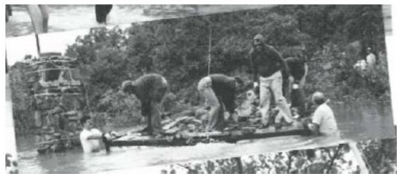
Top: Work crew putting rocks on the pavilion roof of pavilion before second the level addition.
